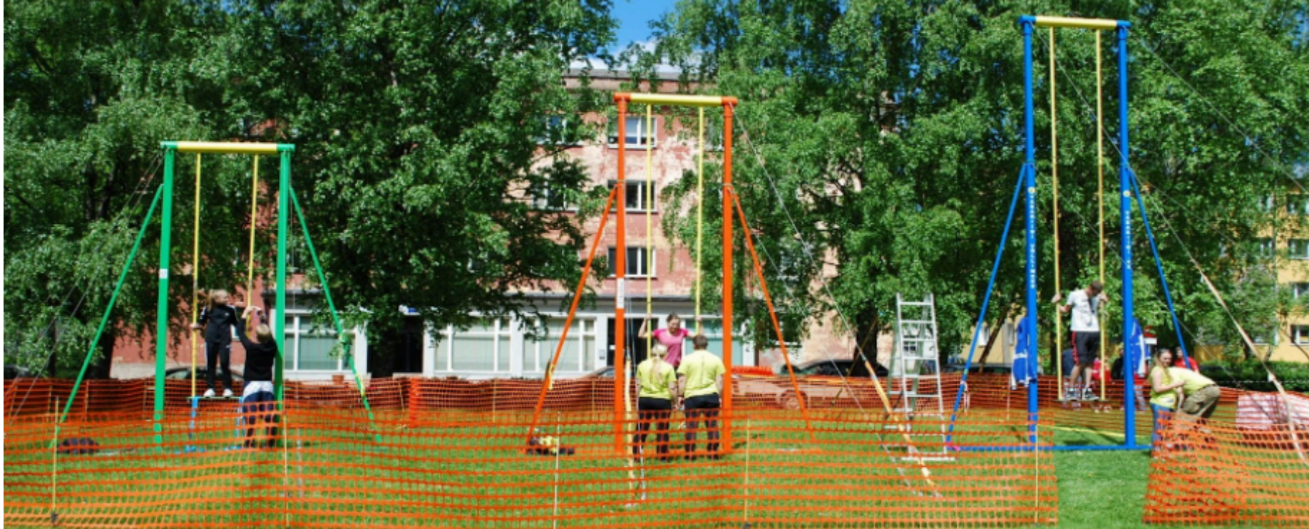
Image 1: Kiiking swings and adjustment interval: KIKI-1(green) 3-4m, KIKI-2(orange) 4-6m, KIKI-3(blue) 4-6m & 6-8m
